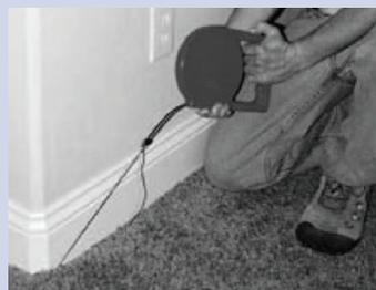
**Figure 4.** Pulling the loop wire up after it has been run under the carpet.
